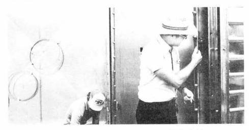
LEAK TEST PORT on inner door seal is checked by TRUPACT Project Leader Vern Romesberg (6322). Outer door behind him has same construction as the outer steel box — a steel tube framework covered on the outer surface with stainless steel sheet. Inside the frame, layers of Kevlar (like that used in bullet-proof vests) and stainless steel serve as puncture shields.
